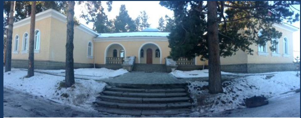
Main building today
